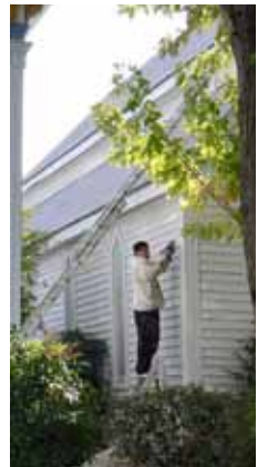
In 2011 we painted the church and replaced the deteriorating cross
